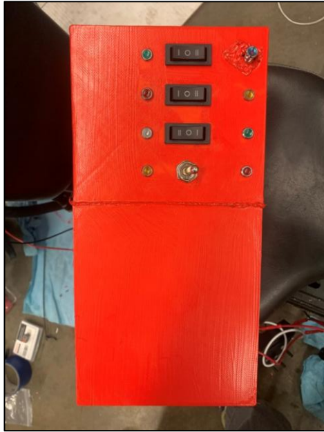
Figure 8: Control Panel and Switches Front View
