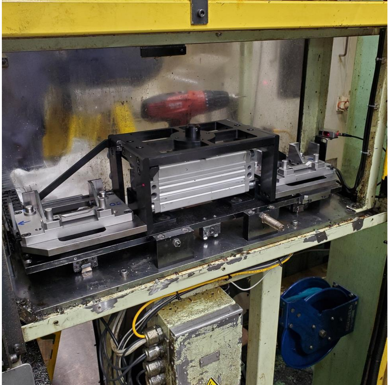
Figure 38 New Infeed Installed
