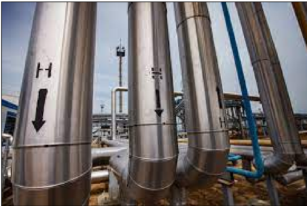
Figure 2-2: Hydrogen Transportation Through Pipelines [11]
