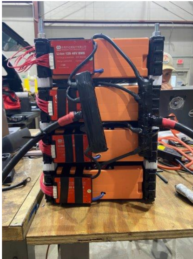
Figure 38 Finished Battery Modules
