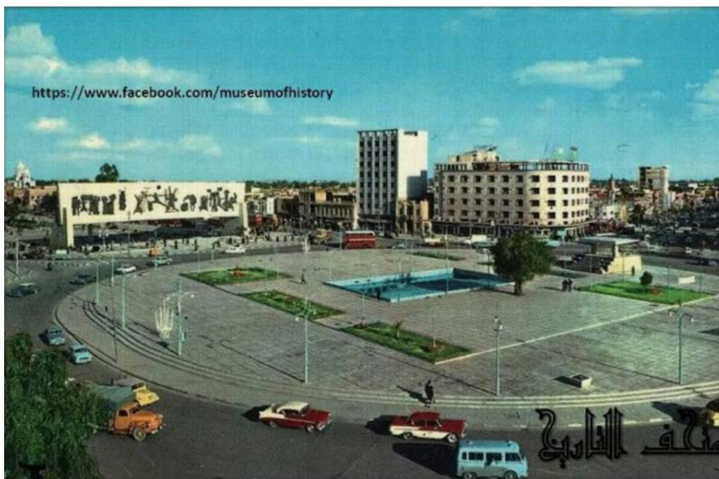
Figure 33: Al-Tahrir in 1963 post-establishment of the Freedom Monument but before construction of the tunnel
