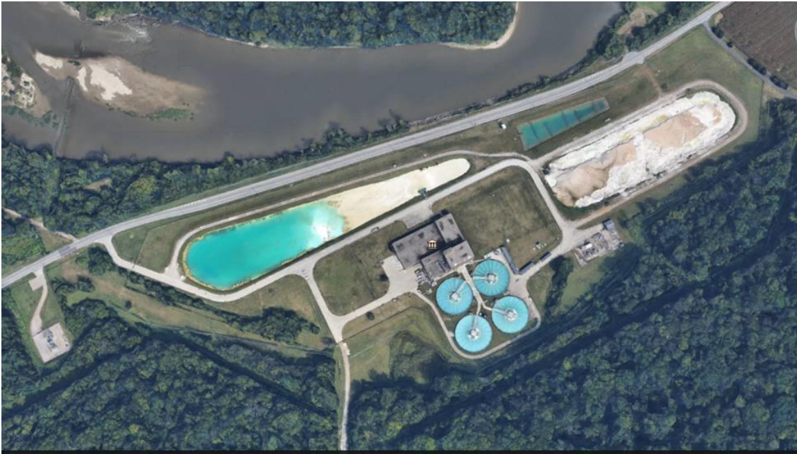
Figure 1. CMBP treatment plant site view
