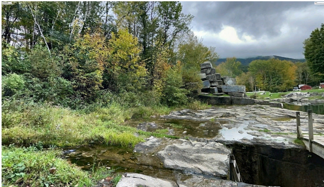
(ABOVE, B7) GOOGLE EARTH, STREET VIEW, DAVID BELL, SEPTEMBER 2022, CARVED OUT MIDDLE SECTION.
