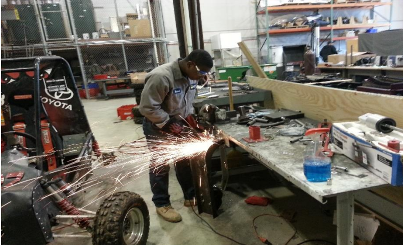
Figure 15: Grinding excess weld beads at steering column
