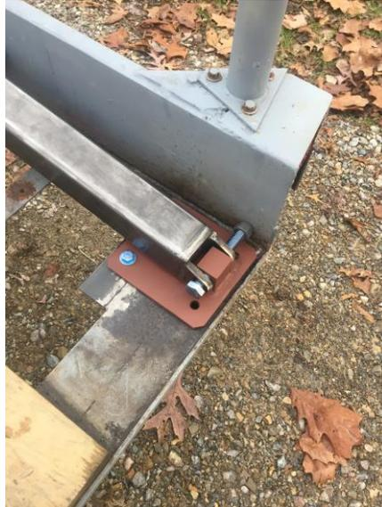
Figure 23: Installing the hinge plates to the trailer framing
