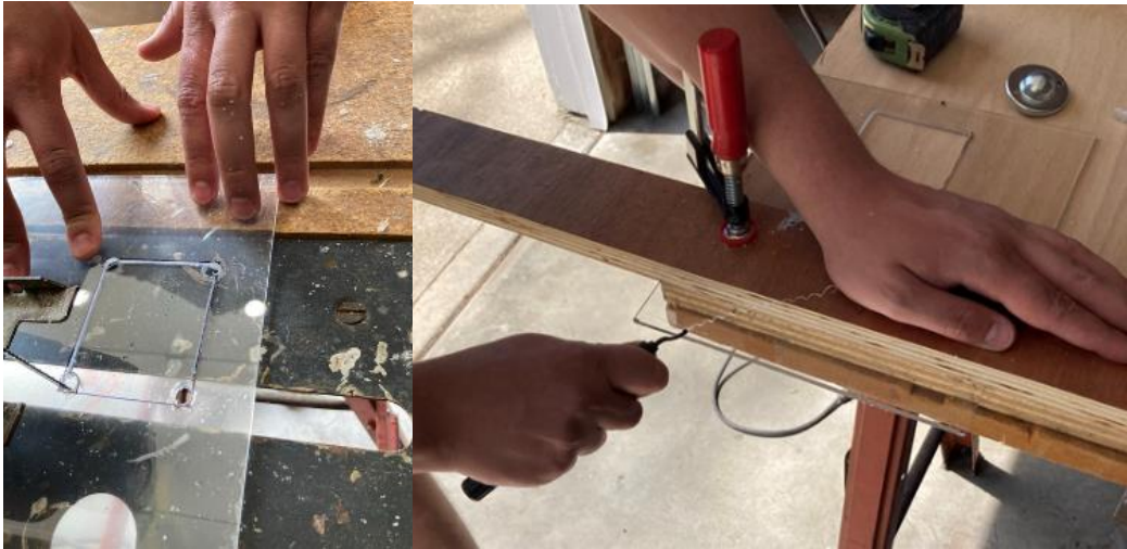
Figure 48: Polycarbonate Wedge Fabrication
