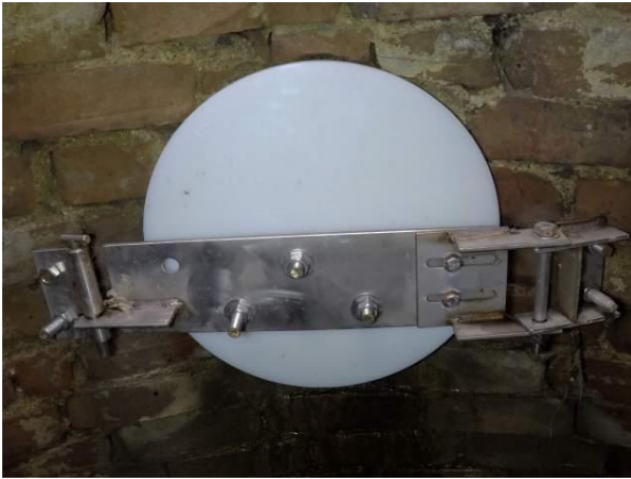
Figure 10.5.2: Coverage Door with 100% coverage
