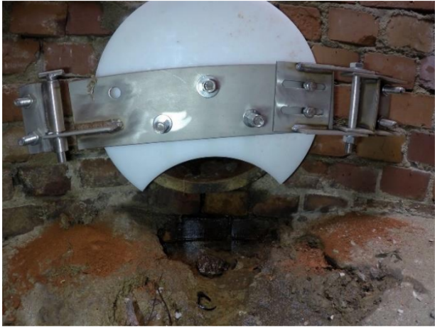
Figure 10.5.1: Coverage Door with opening
