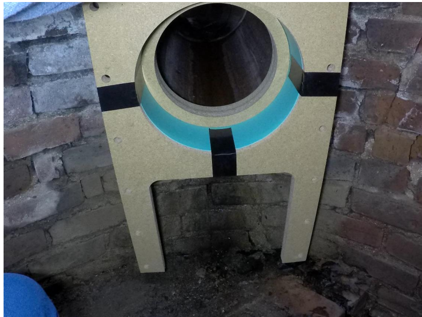
Fig. 2. Beginning of construction of the float control in manhole.
