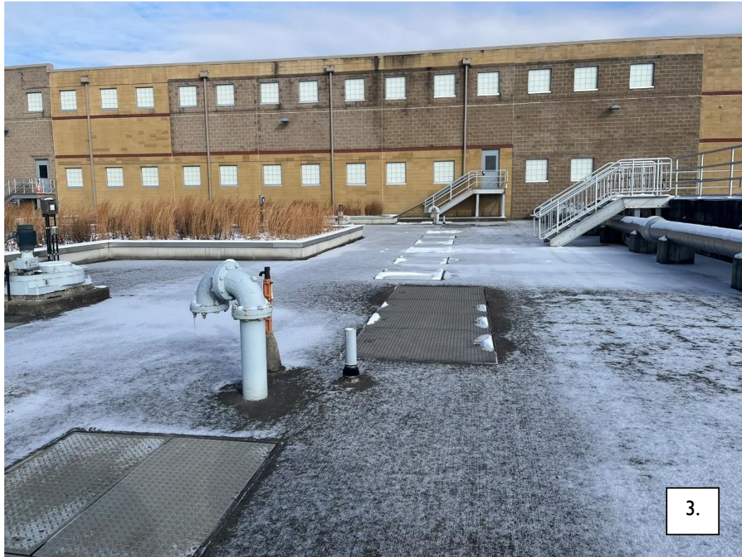
Figure 16, Northern facing view of Green Roof Taken by Annie Lewis 1/20/24
