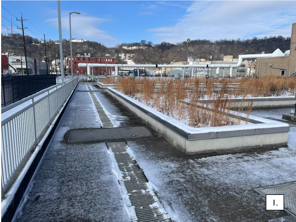
Figure 13, Western facing view of Green Roof Taken by Annie Lewis 1/20/24.
