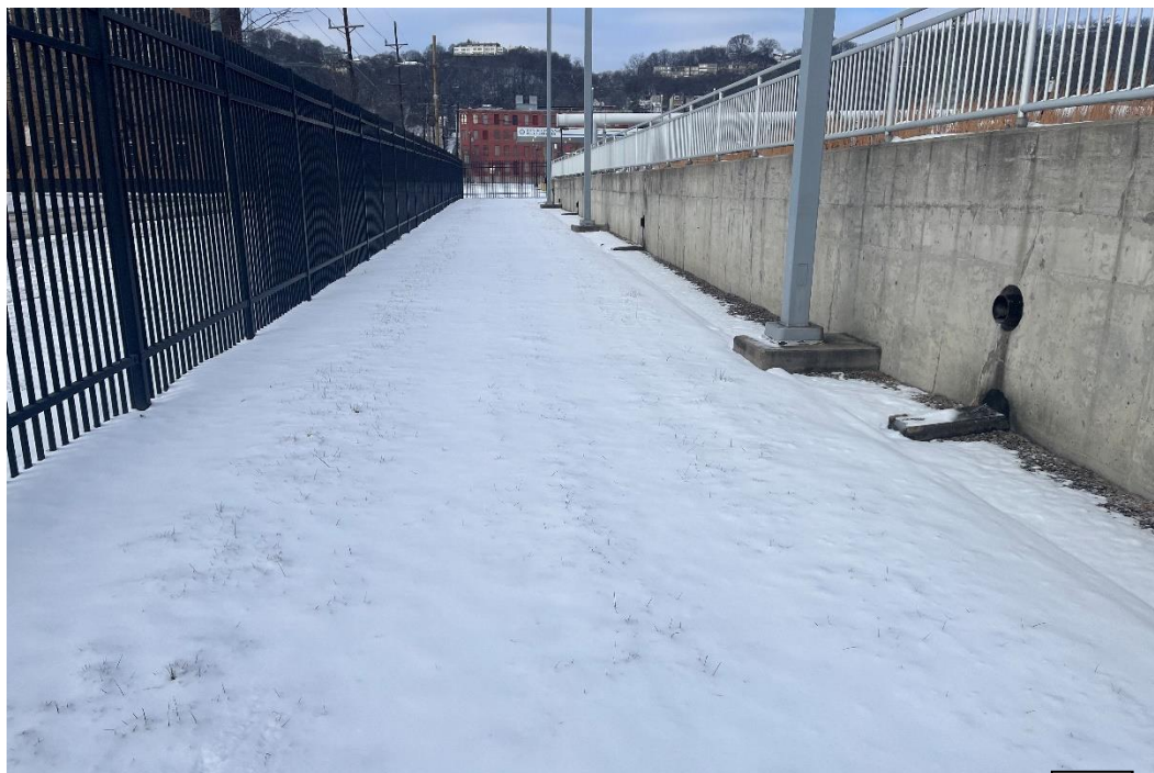
Figure 15, Western facing view from Ground Level of Grit Building Taken by Annie Lewis 1/20/24
