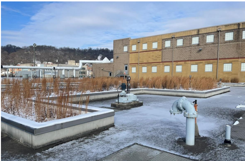
Figure 14, Northwestern facing view of Green Roof Taken by Annie Lewis 1/20/24
