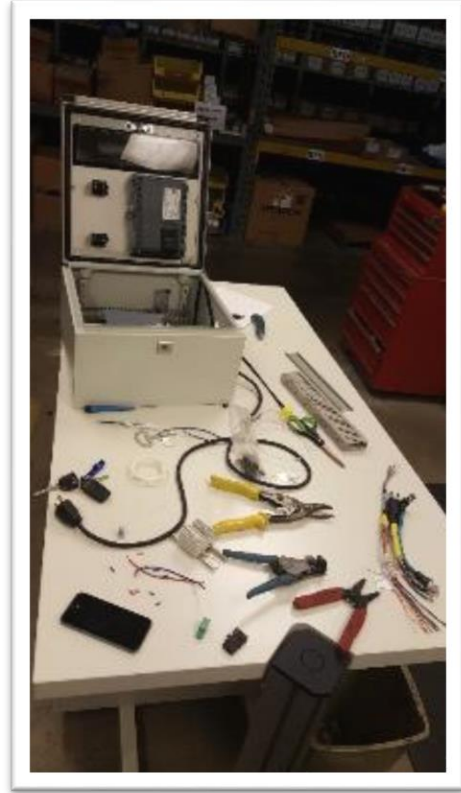
Figure 11: Electrical Enclosure Assembly
