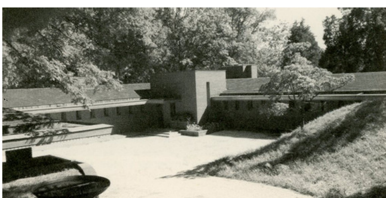
Boswell House, view of entry courtyard, from the north-west. Photograph by Eugenio and Antonella Basan.
