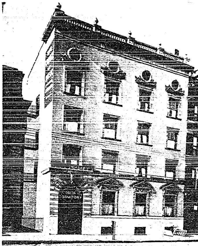
Figure 7.-- Photograph of the Schmidlapp Dormitory, on Elm Street, Taken in 1902.
