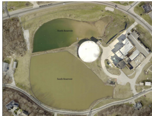
Figure 1: Overview of the Memorial Parkway Treatment Plant
