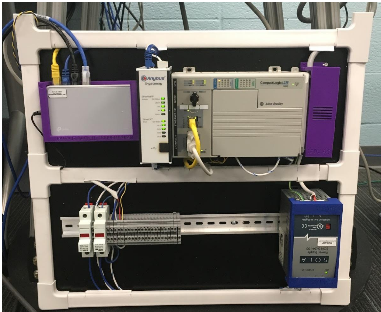
Figure 11A: Main Control Panel Layout
