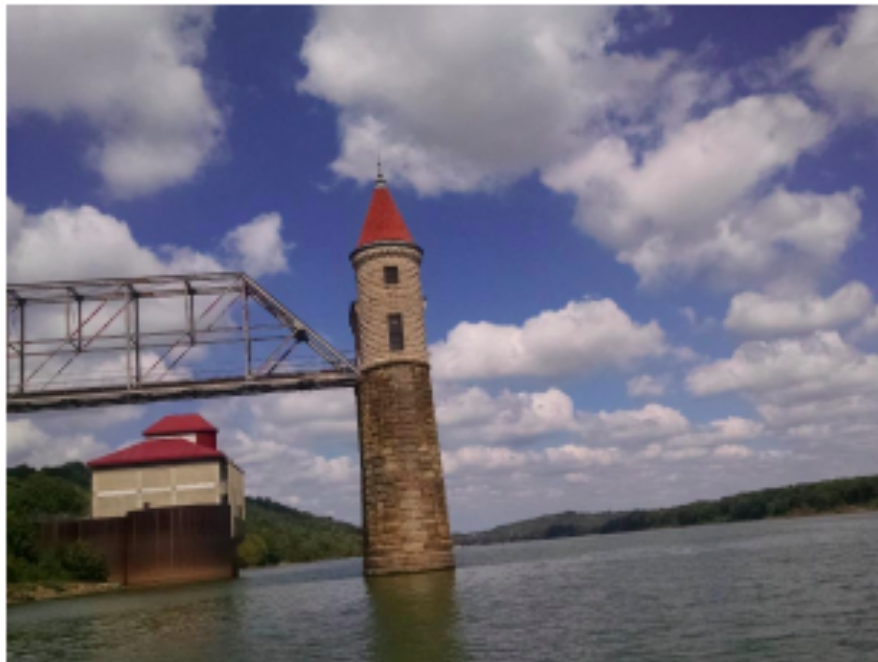
Figure 5. GCWW Intake (foreground) and NKWD Intake (background)
