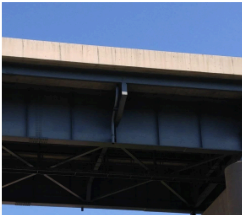
Figure 3. Example of Current Downspout and Storm Water Drain
