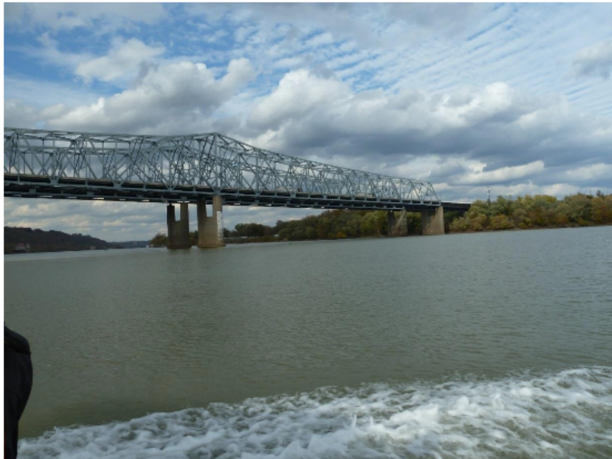
Figure 1: Combs Hehl Bridge located on I-275, California, OH
