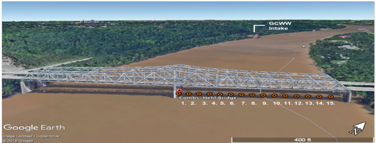
Figure 9: Downspout locations 1-15 along Combs-Hehl Bridge
