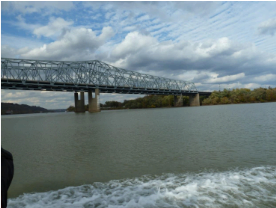
Figure 2. Combs-Hehl Bridge with GCWW and NKWD intakes in left-center of picture
