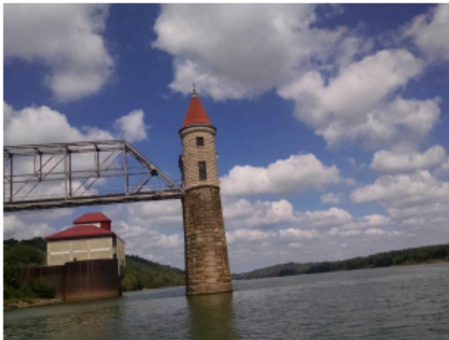
Figure 5. GCWW Intake (foreground) and NKWD Intake (background)
