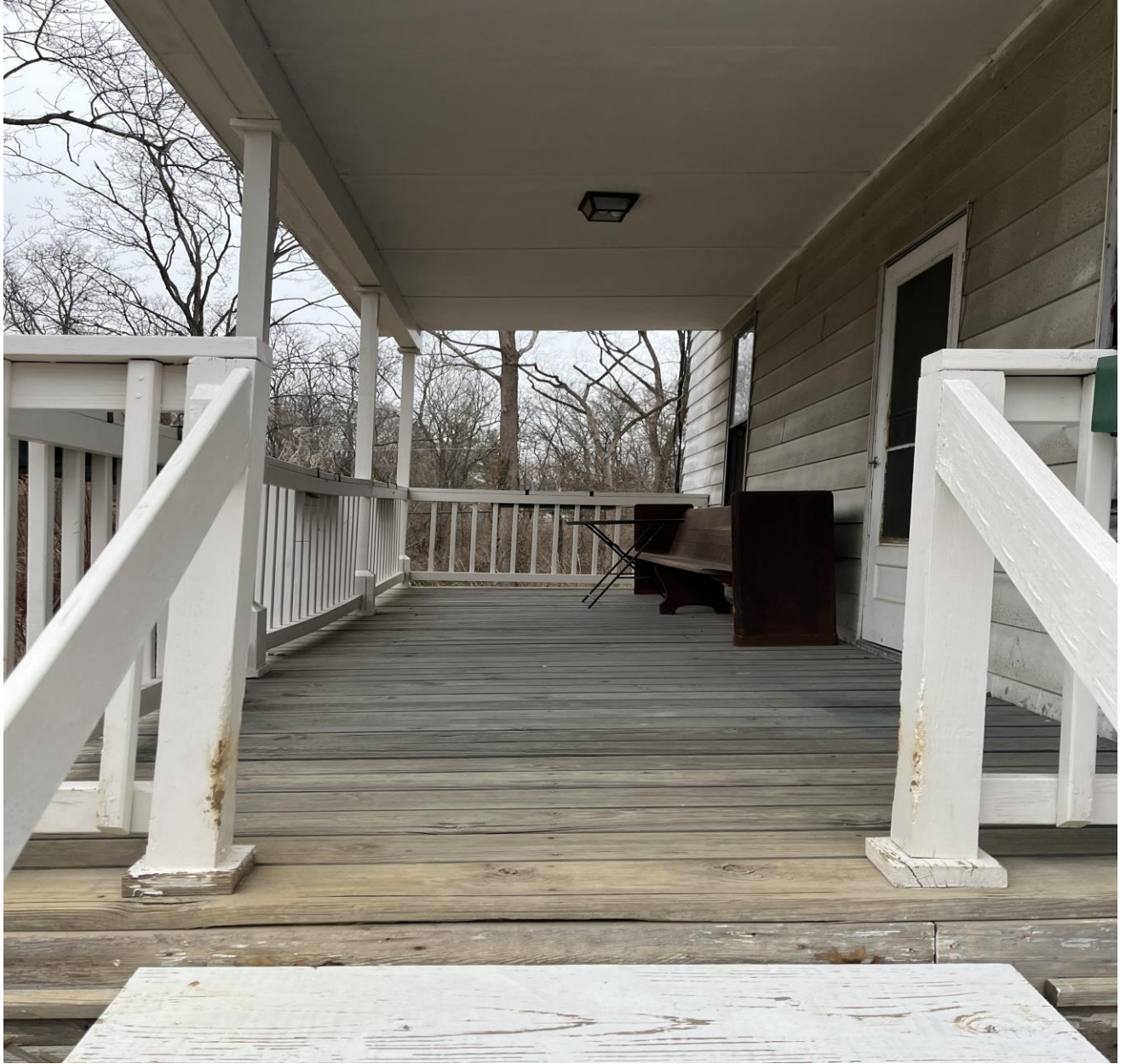
Image 15: Porch on farmhouse. Image Credit: Ben Gressle
