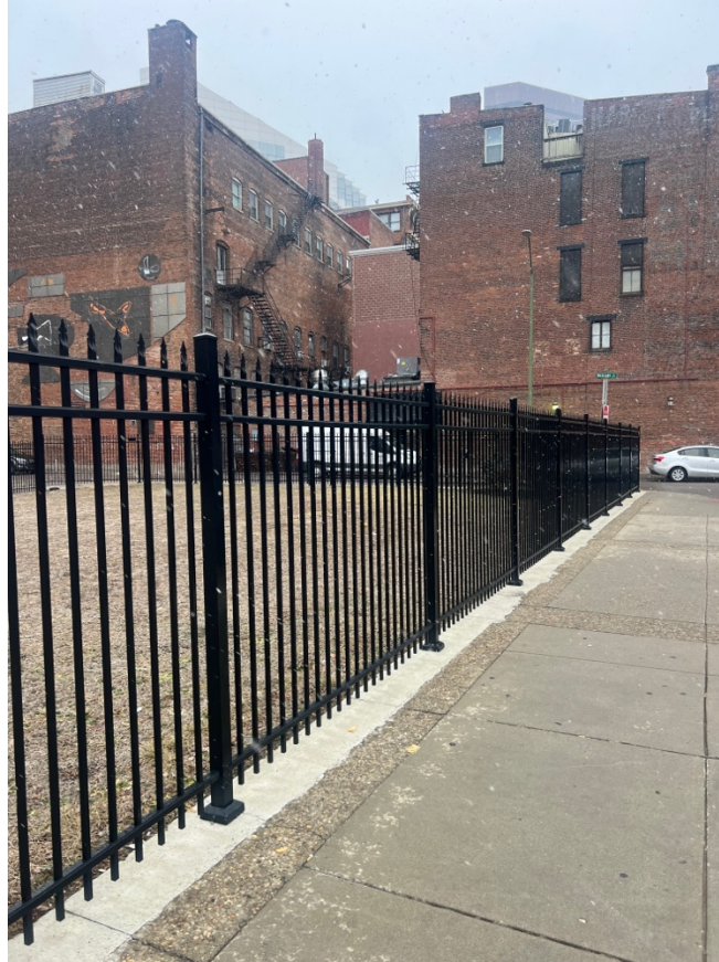
Image showing gating around site.
