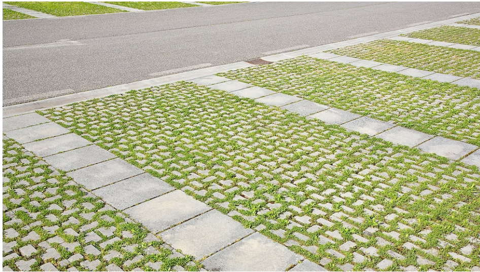
Image of permeable pavers, the ground cover used in the garden design. They are good for managing storm water runoff, reducing erosion, and are ADA-compliant.
