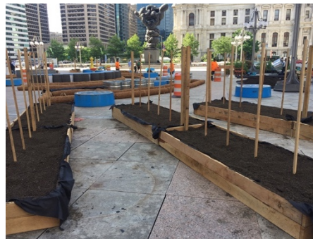
Image showing renewable materials used on-site. The image shows components of the farm that were built off-site and installed in one week.
