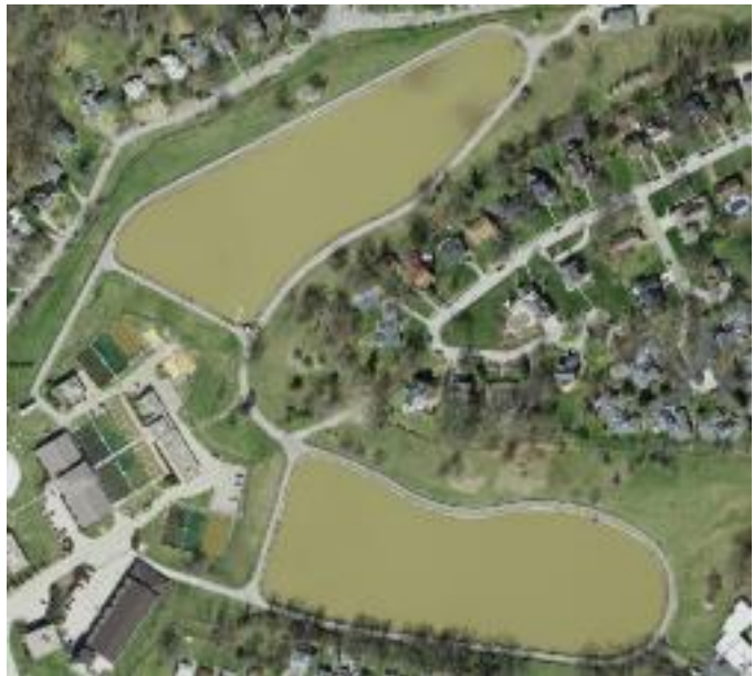
Figure 2: Fort Thomas Treatment Plant
