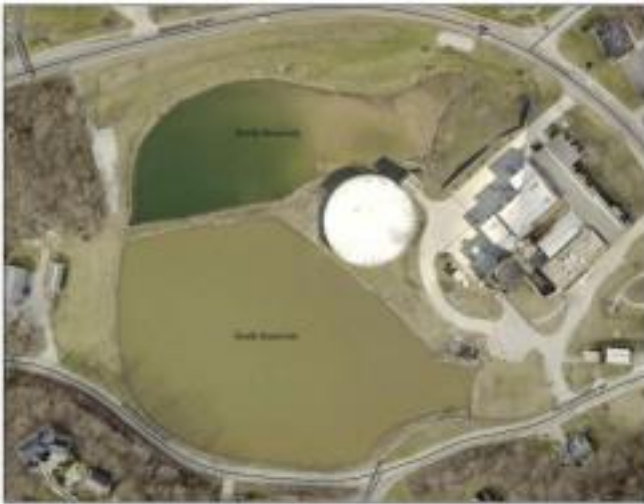
Figure 1: Memorial Parkway Treatment Plant
