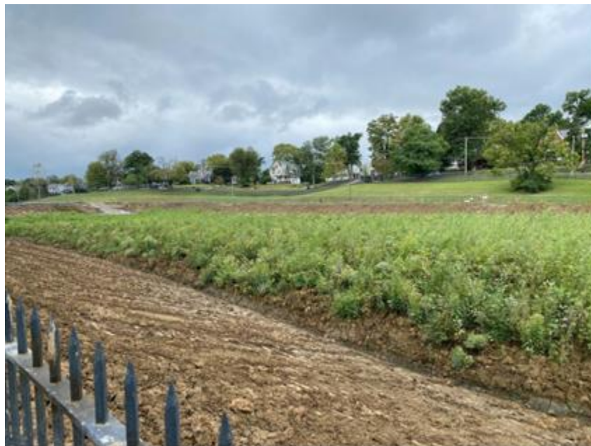
Figure 1-2: North Reservoir at FTTP (9/21/21)
