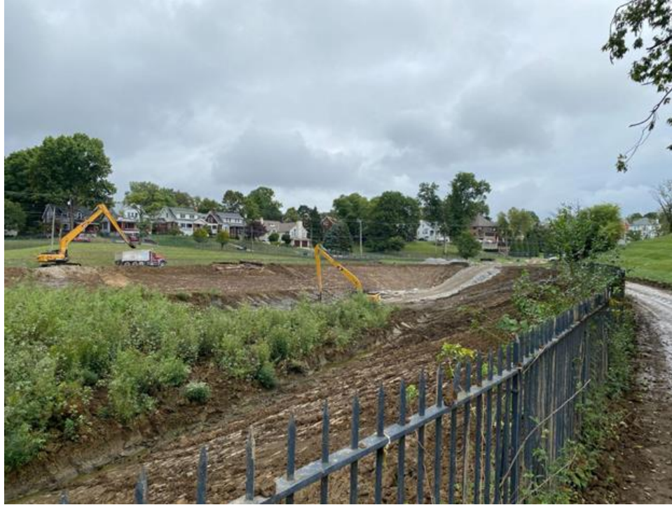
Figure 2-6: North Reservoir Excavation (9/21/21)
