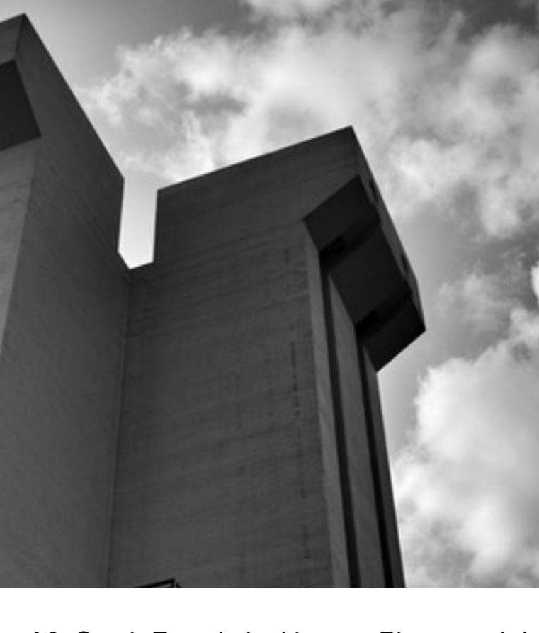
Crosley Tower | Building A2, Detail of East Façade. Photograph by Elizabeth Meyer
