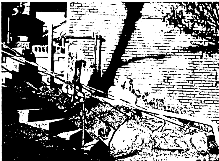
Figure A.8 Water main break at the West View Condominium. The water main break caused the ground adjacent to the building to drop several inches and the down slope soil to bulge.
