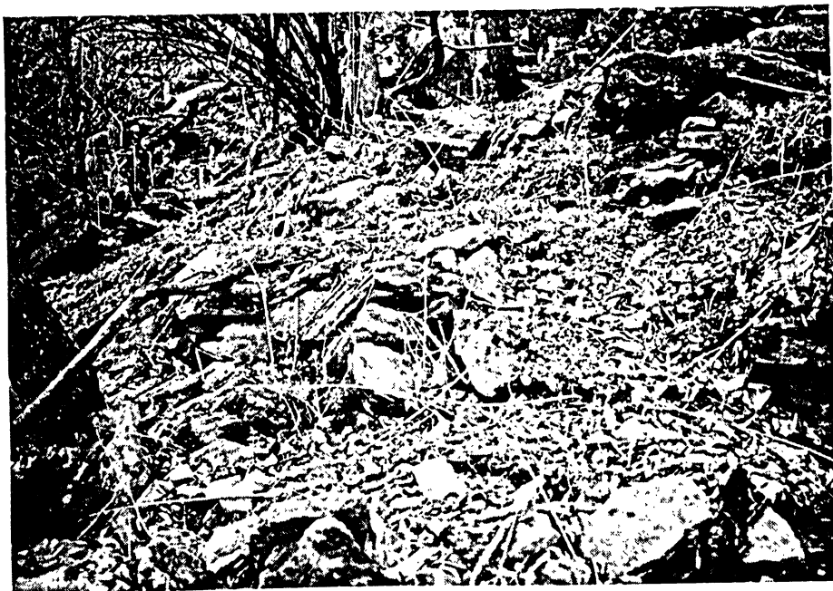
Figure D.24 Limestone rubble pile located midslope.
