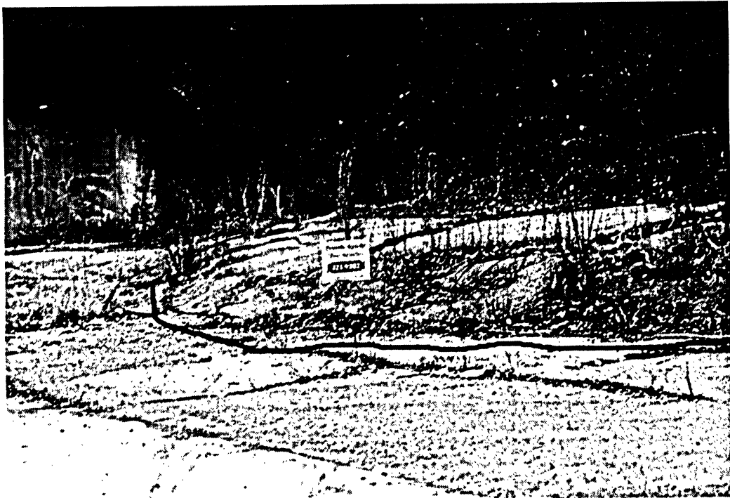
Figure D.4 Landslide toe located off of River Road in asphalt parking lot. Illustrates subtle nature of uplifted toe area, readily apparent because it crosses man-made feature. Real estate sign is eighteen inches high.
