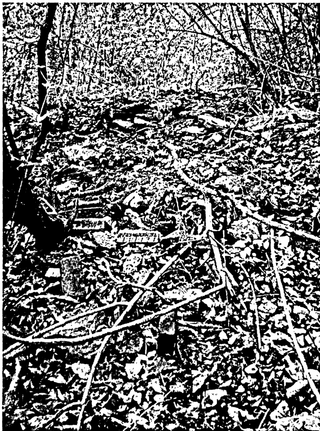
Figure D.30 Limestone rubble and paver brick used as road base for Rudolph Avenue.
