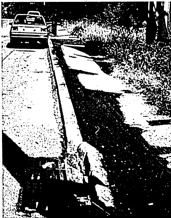
Figure F.13 Warsaw Avenue in 1992 prior to pier wall correction project by the City of Cincinnati. Disheveled nature of the sidewalk is indicative of landsliding. The ground surface below Warsaw Avenue in this area is indistinct. Photograph courtesy of the City of Cincinnati.
