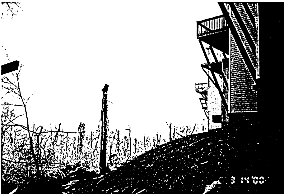
Figure D.22 Clear cutting and topping of trees for the view. Note that deck supports are braced against the foundation.
