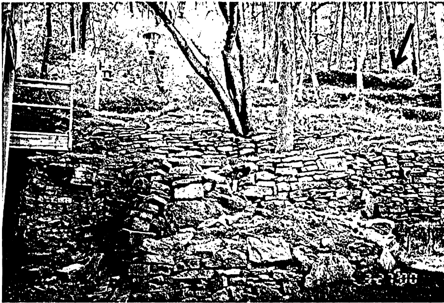
Figure D.21 Series of limestone walls just above Maryland Avenue. Goforth Avenue terrace (arrow) as seen looking west from Maryland Avenue.
