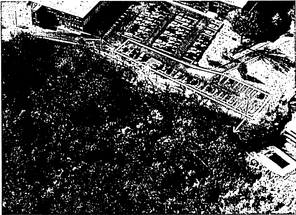
Figure F.14 Oblique aerial photograph of the Cincinnati Bible College parking lot and hillslope above Neff Street. A large portion (area outlined in white) of the parking lot drains down the hillside onto a highly disturbed area. Note the pier wall in front of the building in the upper left corner of the photo. Also note the swimming pool for an apartment building in the lower right corner empties onto the hillslope.
