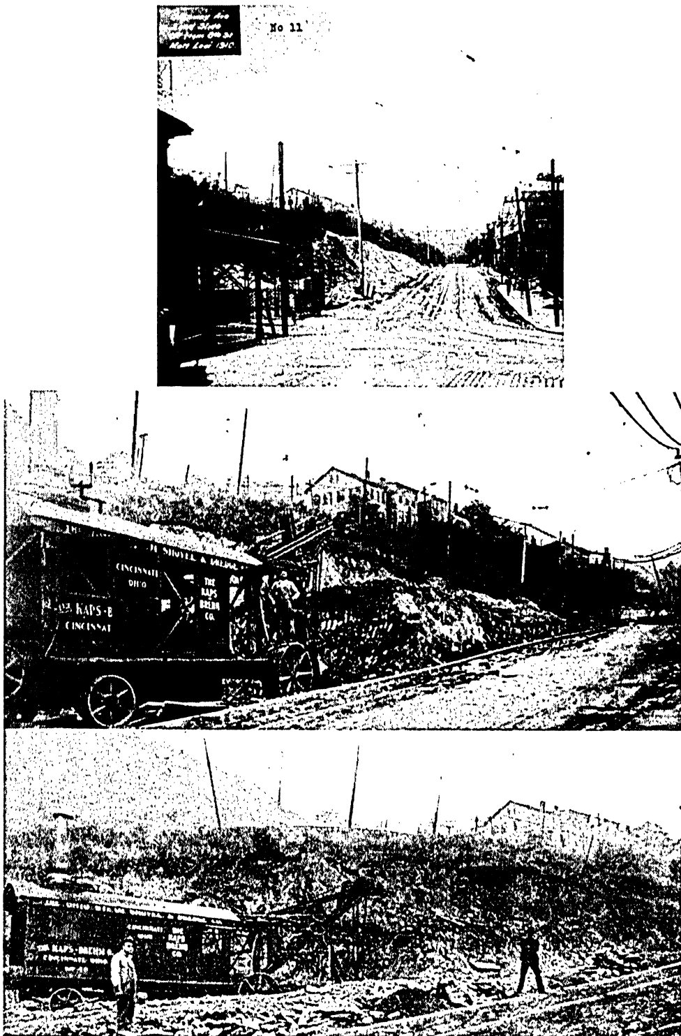
Figure F.7 Upper photograph (1910) shows toe of landslide on Glenway Avenue just north of the Incline. Lower two photographs (early 1900's) show the widening of Glenway Avenue and the toe of the hillslope and/or the landslide mass being excavated below the bend in Wilder Avenue. From the Cincinnati Historical Society collection.
