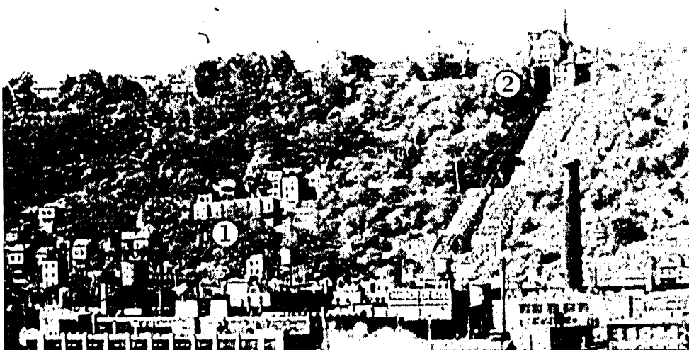
Figure F.10 Area 1 is a buttressed limestone wall above Maryland Avenue and located below the Goforth Street terrace. Area 2 is the Incline house. Photograph courtesy of the University of Cincinnati.
