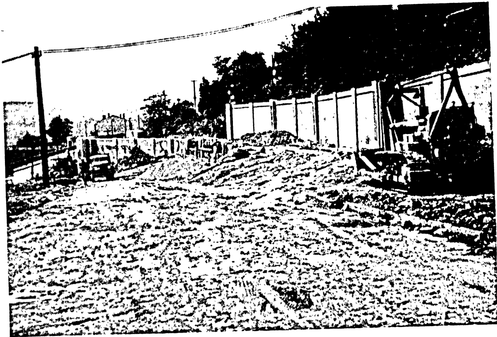
Figure F.4 Construction of the Warsaw-Waldvogel Viaduct in 1950.
