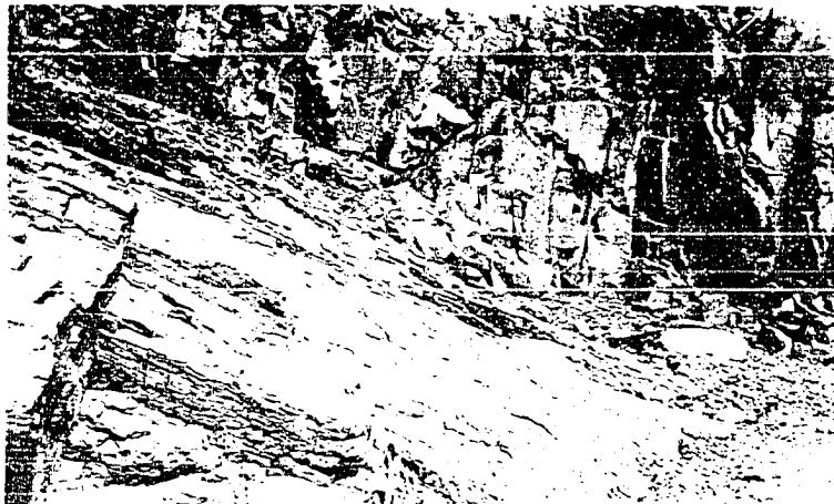
Fig. 5 Looking down on slabby top of a flow from which the dense blocky overlying flow is being stripped.
