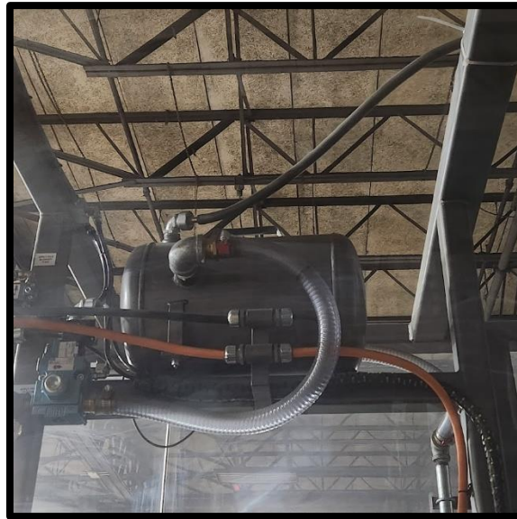
Figure 27 – Air hose connection to vacuum tank
