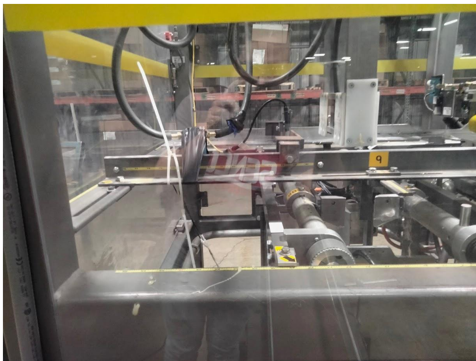
Figure 29 – Air hose connections from vacuum tank to suction cups through the solenoid, machine operator side.
