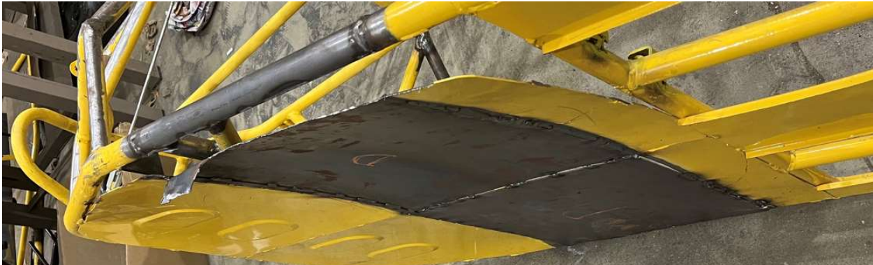
Figure 35: Removal of bottom plate
