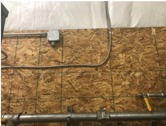
Figure 1.20. the image on the left shows the electrical conduit and electrical box above the existing nitrogen generator. The image on the right shows the conduit and electrical moved.
