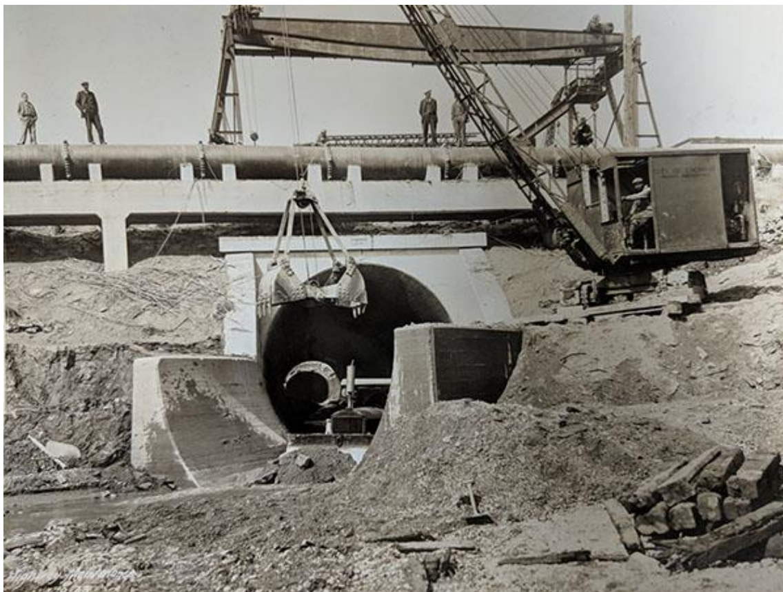
Figure 17. Construction of a combined sewer outfall into the Mill Creek in Cincinnati Ohio, 1933 (Smith, Trail location 8: History of a Watershed n.d.).
