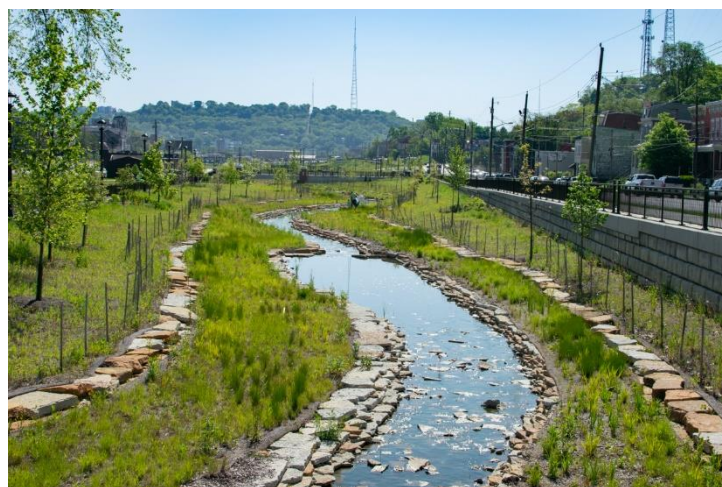
Figure 4. An example of green techniques being implemented to reduce stormwater runoff at the Lick Run project (Smith n.d.).
