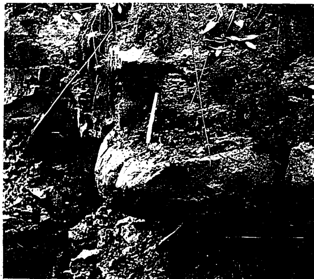
Fig. A8. - Section 1565-CT; Titusville Quadrangle, 20' north of Fig. A7 in a ditch excavated for a water line. The pencil rests upon a massive calcareous lenticle in the basal Corry sandstone.
