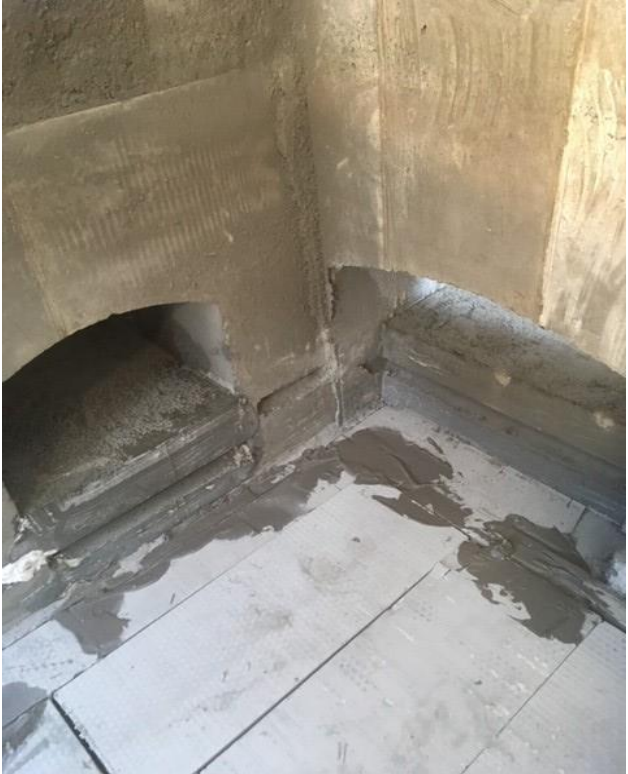
Figure 26 shows the inlet well and pump well from the inside of the holder.
