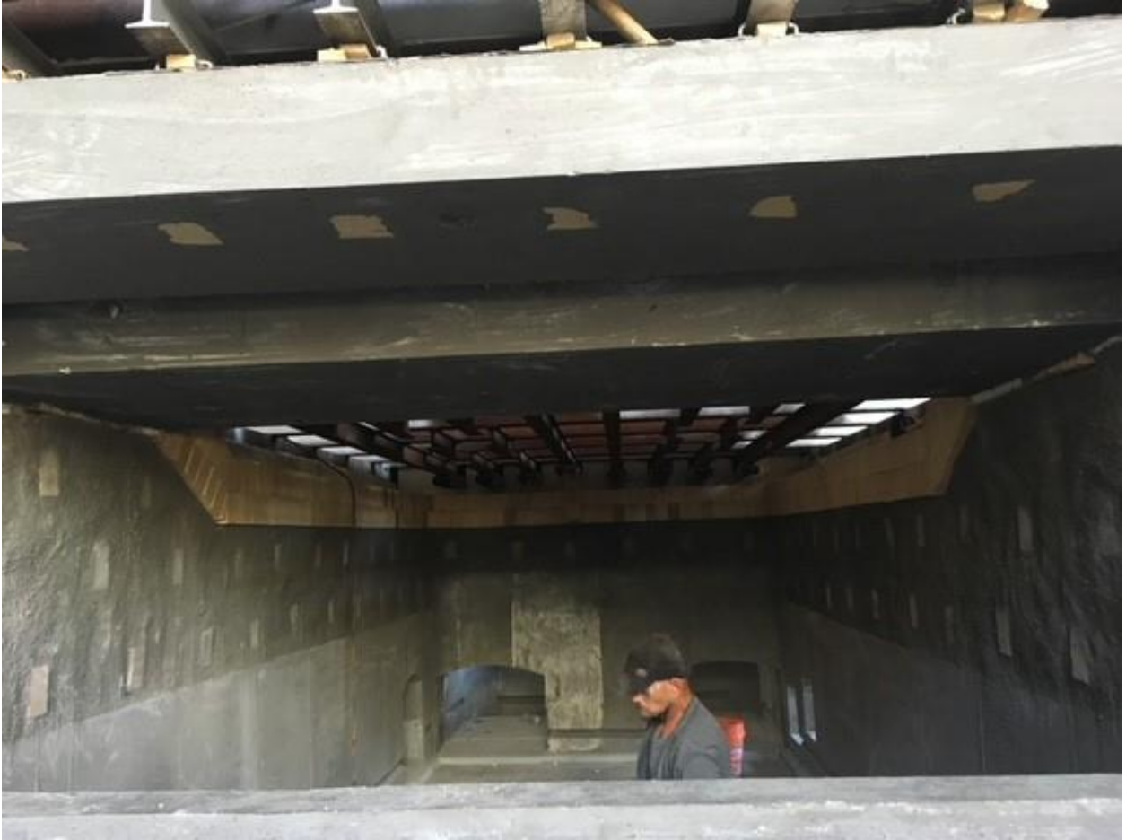
Figure 29 shows the inside of the holder before the roof was built.
